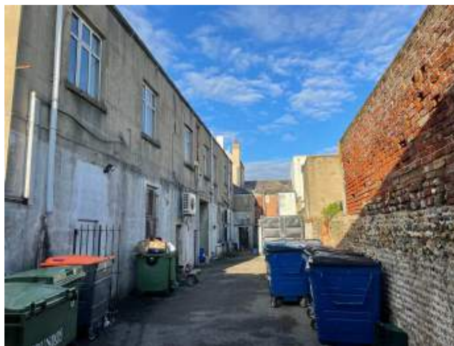
2. Exterior, service yard
