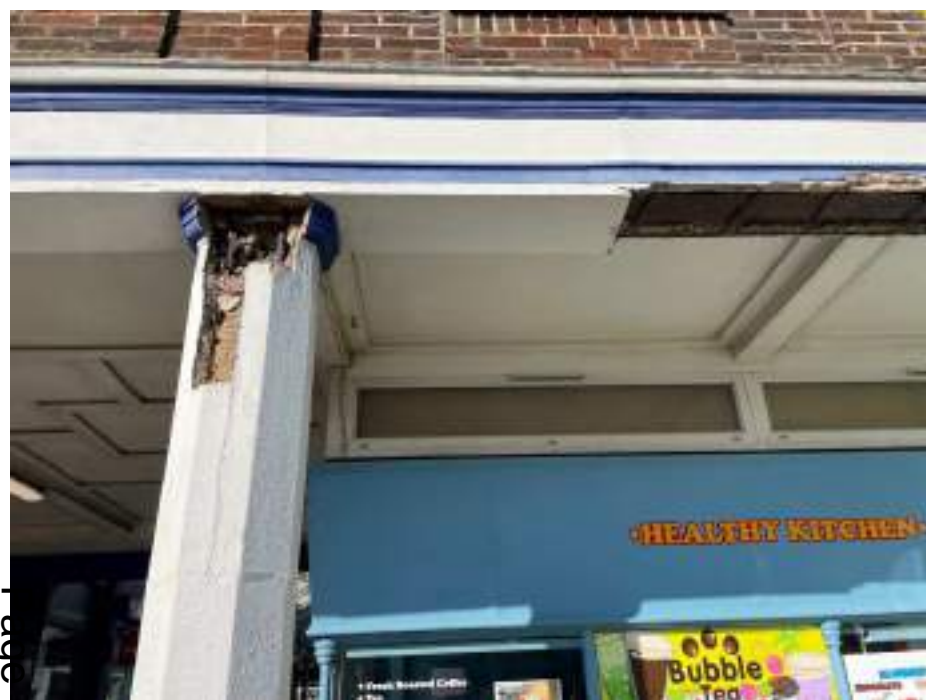
1. Exterior, Belmont Street
